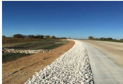
State Roads Route AC Construction in Perry County, MO
