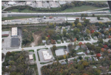
Overlays (Streets & Roads) Merriam Lane Reconstruction & Improvements (24th to 10th Street) in Kansas City, KS
